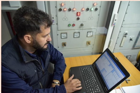
Stefche Stefanovski, head of Relay Protection and Secondary Connection
